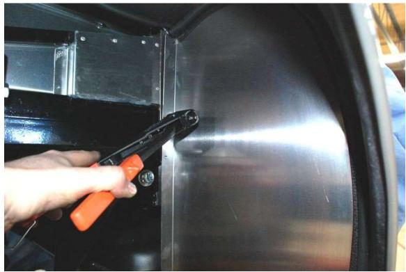
Silicone and rivet the panels in place.
