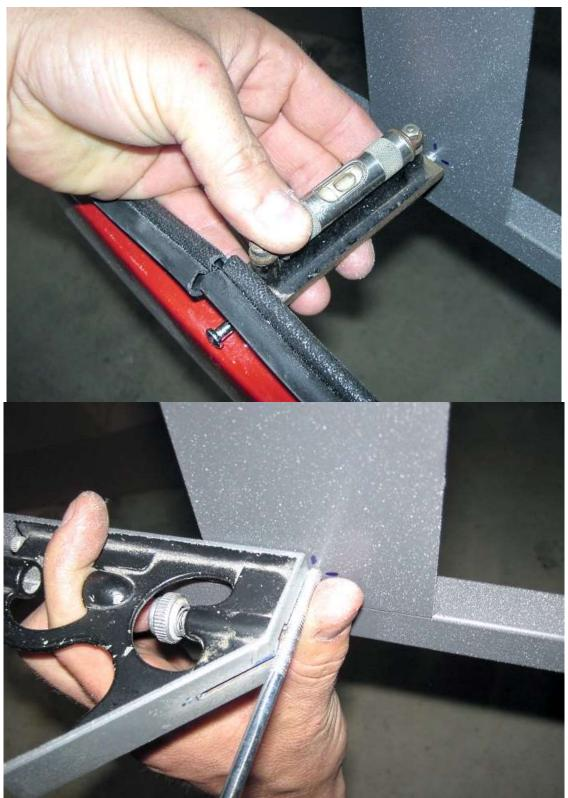
Put the pin screw through the body and up to the frame. Use a level and a square to locate the end of the screw.
