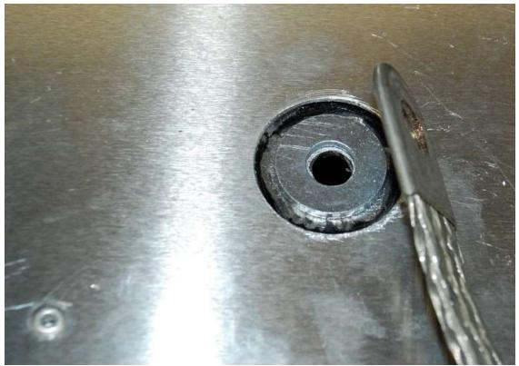
Drill through the center of the circle and put a washer down in the cut out.
