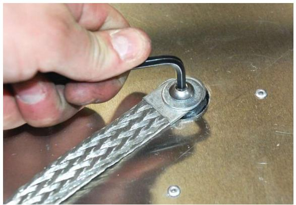
Attach the ground strap to the chassis with the supplied  $\frac{5}{16}$ " button head screw, locknut,  $\frac{3}{16}$ " hex key and  $\frac{1}{2}$ " socket.
